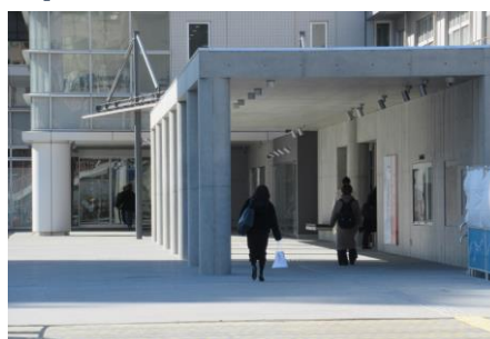
Near the new entrances of City Hall and City Hall Annex
