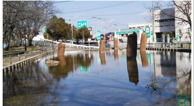
The remains of bridge piers
