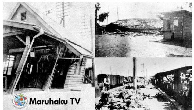
Collapsed Chigasaki Station (Maruhaku TV)
